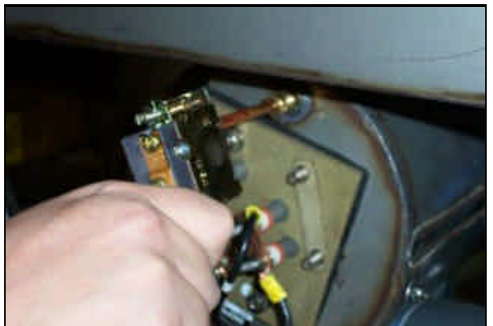
Putting the new thermostat in the well.
